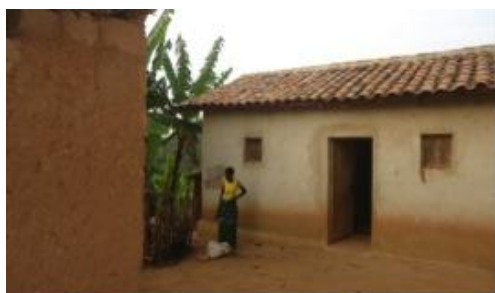
Francine - house now complete with good roof and doors
