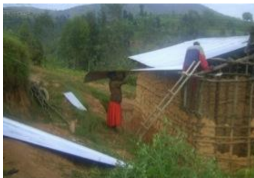
Alvera helping to build her house.
